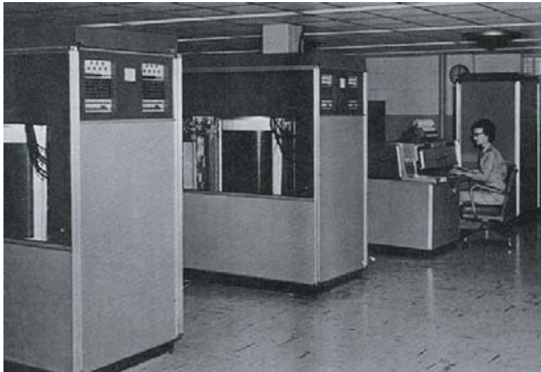
Figure 1.1: The first hard disk drive. [Wikipedia 2010]
